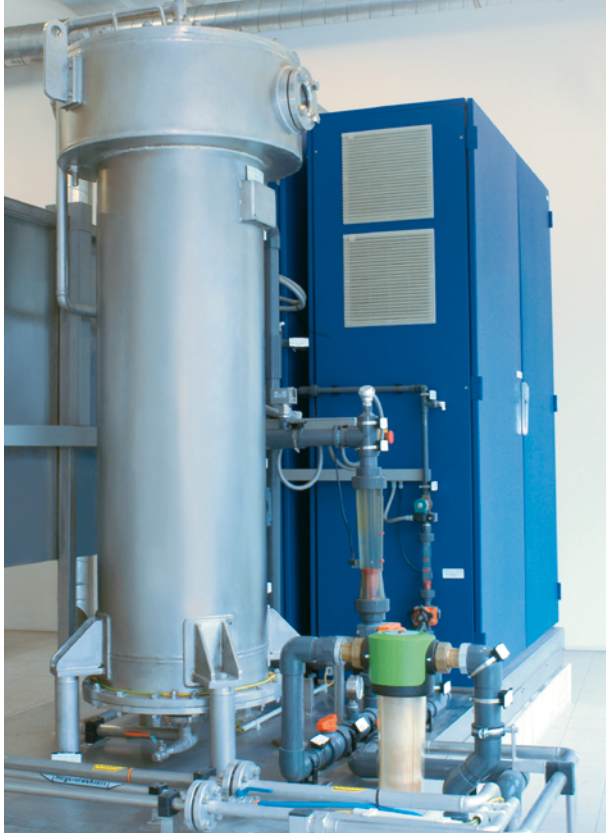
Modern ozone generators, such as this system with a production capacity of 3kg/h, use pure oxygen as the feed gas.
