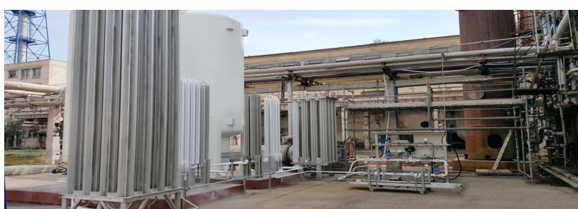
**Figure 4.** Test equipment including a mobile tank, vaporisers, fundaments, regulation skid and flexible hoses.
