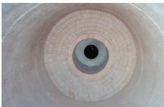
*CLAU S combustion chamber in operation*
